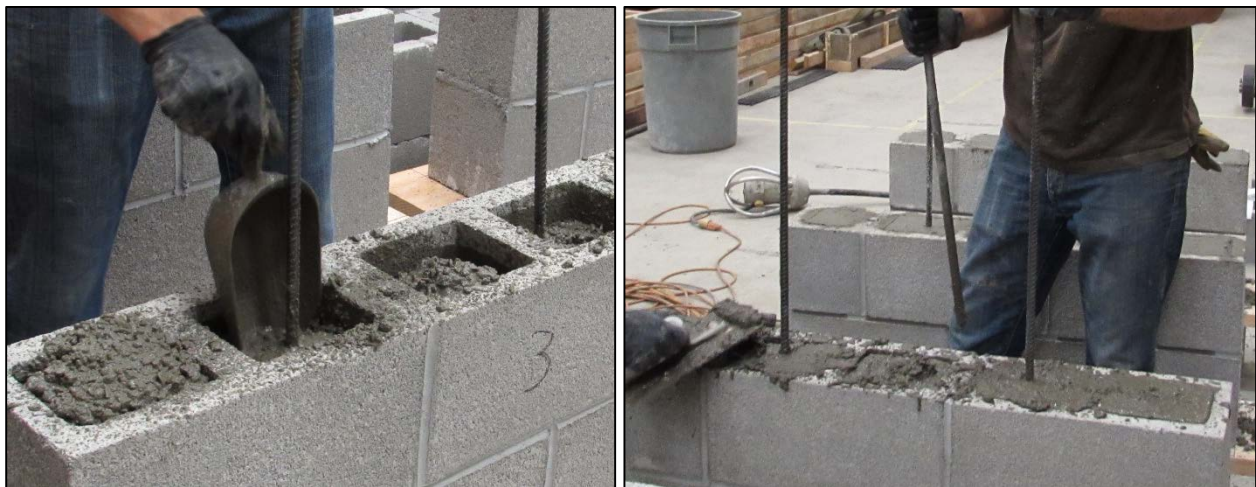
Figure 18. Filling Top Portion of Walette
