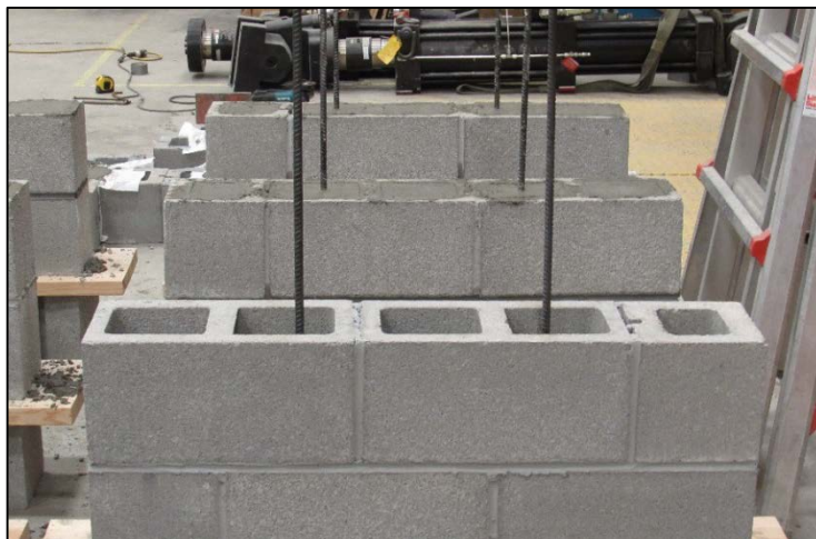
Figure 16. Placement of Reinforcement Prior to Grouting
