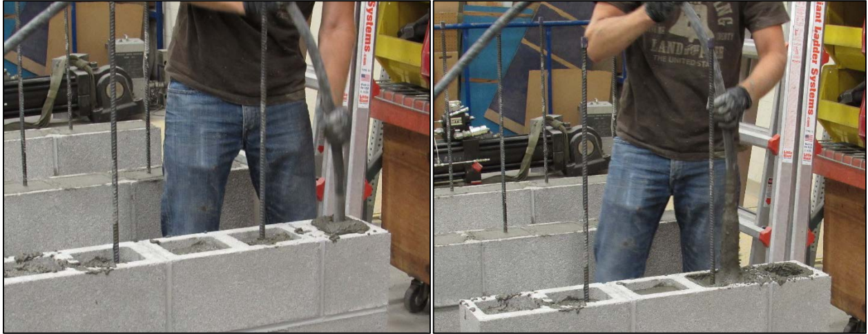
Figure 19. Consolidation of Grout using Vibratory Stinger
