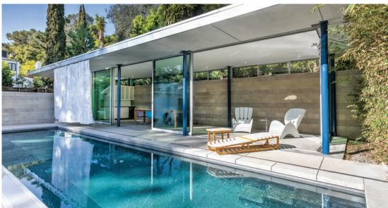
**ARCHITECT'S COMMENTARY:** The pool house and lap pool are an independent addition to an existing California style bungalow. The floating roof is independently supported on eight steel columns. The ribbon of clerestory windows above the concrete masonry unit (CMU) retaining wall reinforces the visual sense of the floating roof. The lap pool reinforces the horizontality of the floating roof and is heated by an array of solar collectors, which provide 100% of the heat during the summer months.
