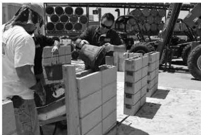
Figure 4: Bucketing Grout into Sample Panel
