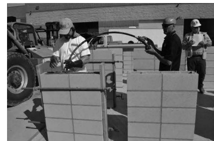
Figure 5: Consolidating Grout
