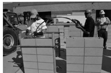
Figure 5: Consolidating Grout
