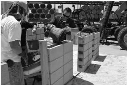
Figure 4: Bucketing Grout into Sample Panel
