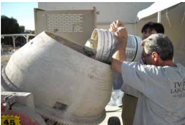
Figure 1: Adding Grout Materials to a Mechanical Mixer
