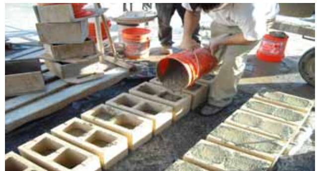
Figure 2: Grout Placement in Concrete Masonry Unit Cells
