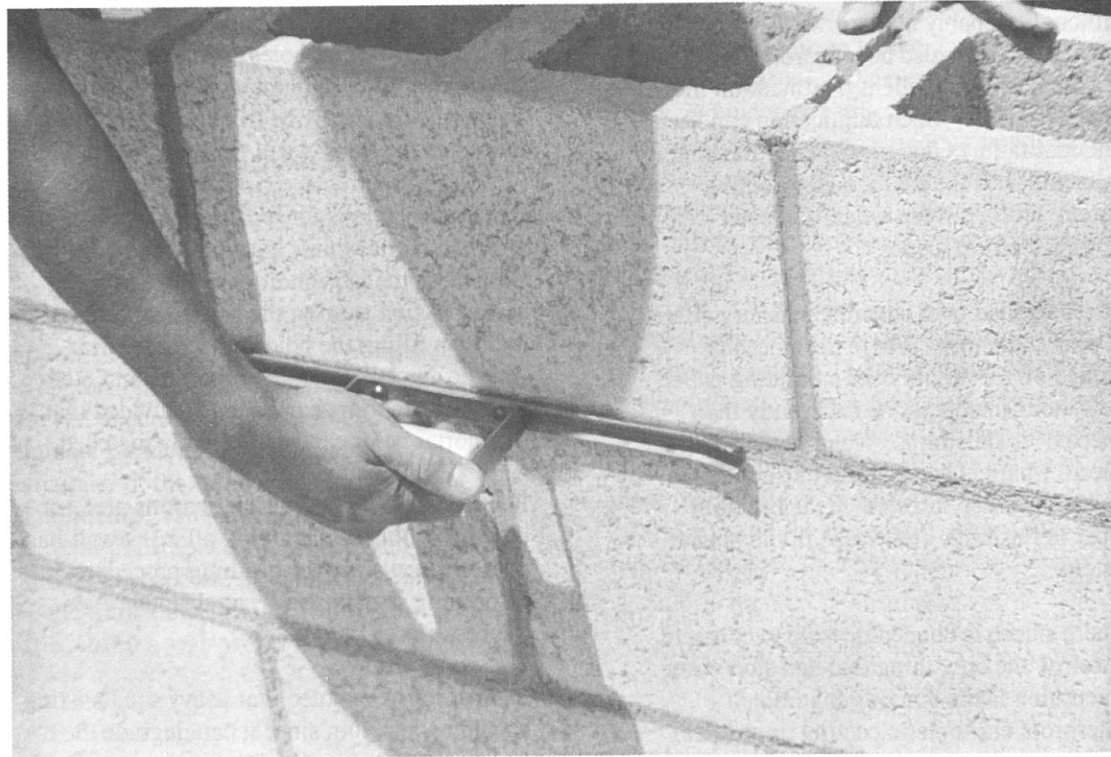
Concave tooling of mortar joints with a sledrunner tool.
