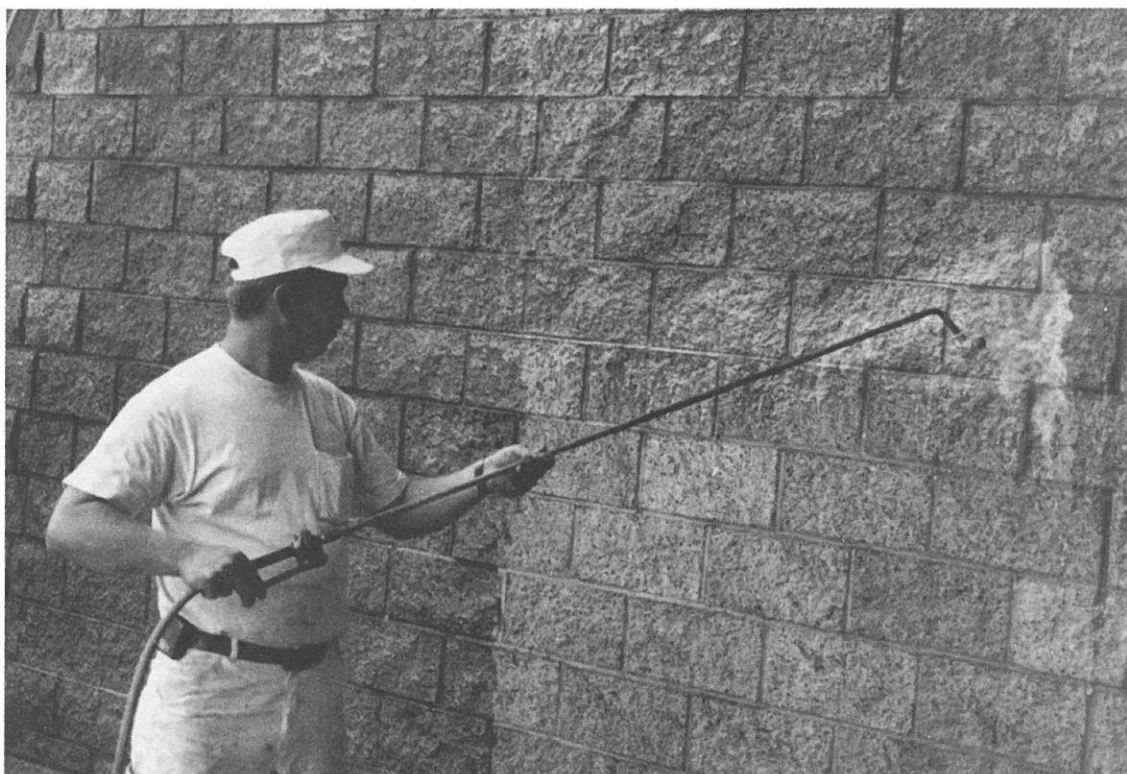
Application of clear water repellent on split face concrete masonry wall.
