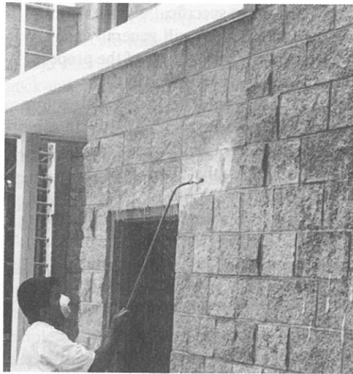
Spraying water repellent chemicals on split face concrete masonry wall.
