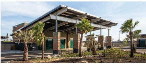
WHY MASONRY? The area around the project site has mostly aging tilt-up concrete buildings. Concrete masonry units (CMUs) offered a structural material with a great variety of options for color and finish texture, which allowed for an aesthetically pleasing durable building to be constructed well within budget.
