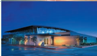
ANGELUS BLOCK HEADQUARTERS SUN VALLEY, CALIFORNIA
