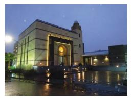
Why Masonry? The program guidelines provided to the design team included a requirement for longevity of the mosque structure. The other critical guideline was to ensure that the building stay cool and allow for air-movement. Selection of 12" thick concrete masonry units for the main prayer hall building became a natural choice, the stone cladding allowed the structure to reflect the traditional color palette on the exterior face and furred construction allowed for additional thermal insulation.
