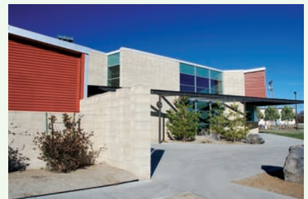
©Photography: Angela Bigotti, AIA, large photo and insets 2 and 3 Greg Anderson, Greg Anderson Photography, inset 1
