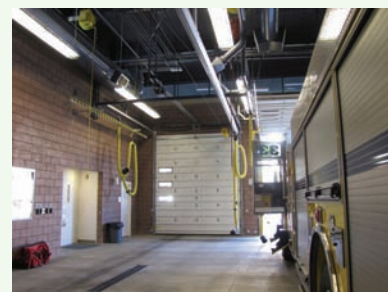
Photography: Shaun P. Yauch, AIA, BJG Architecture + Engineering
