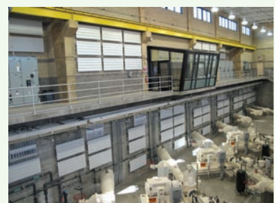
Photography: Greg Gould, Carollo Engineers
